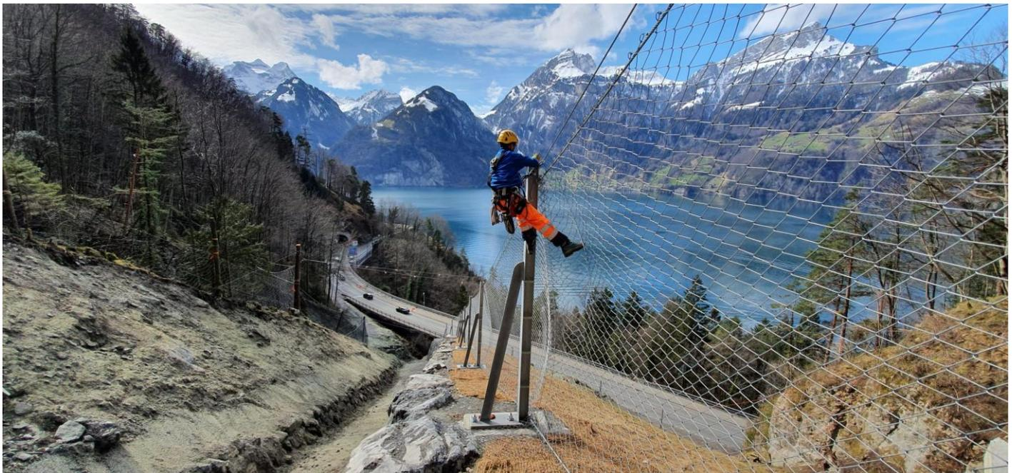
Figure 2: Installation of motion sensors on the high-tensile steel flexible rockfall protection barriers installed on the deflection dam.
