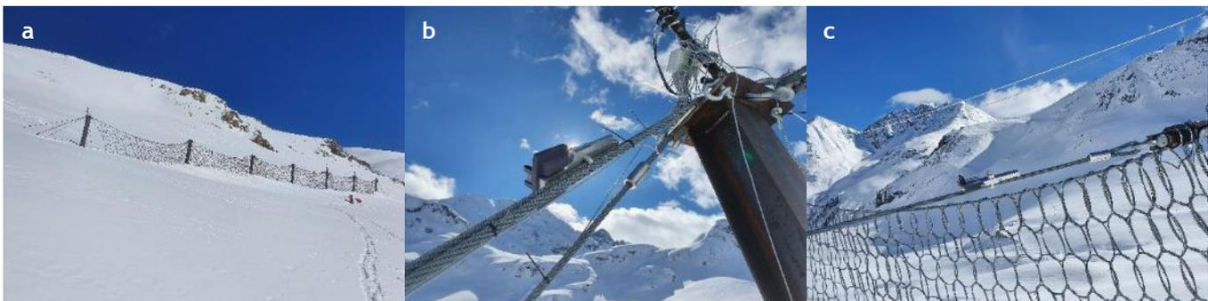
Figure 2: a: barrier embedded in snow; b: detail on measuring equipment at post head such as rope forces; c: digital device monitoring the barrier's state
